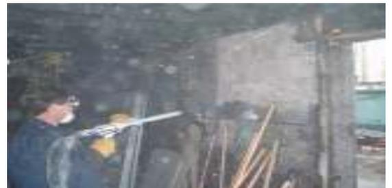
*Above: Removal of soot from concrete block wall*
